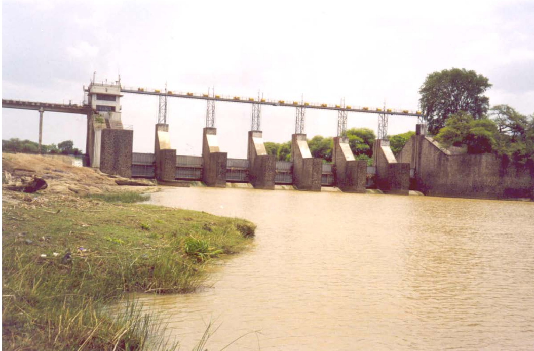
Figure 1: Gated spillway for controlled water discharge.
